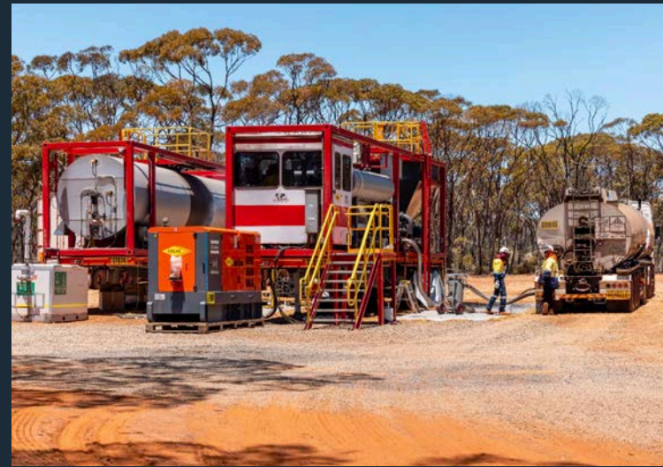
Mobile CRMB blending plant in operation in the Pilbara region
