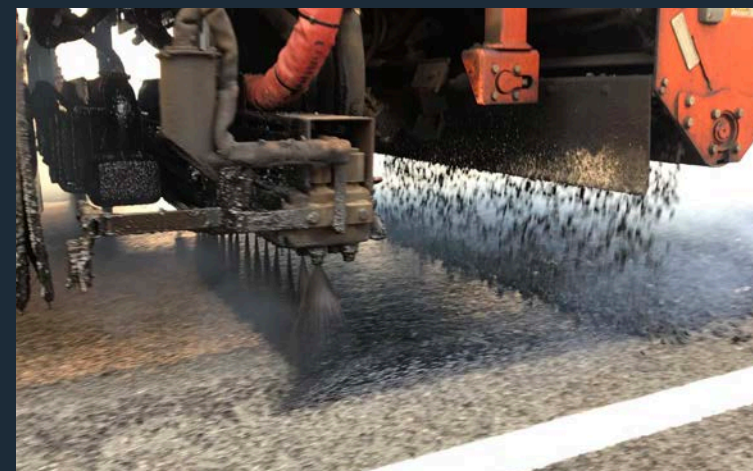
LV S15R being sprayed by the OB Vario synchronised sprayer and spreader
