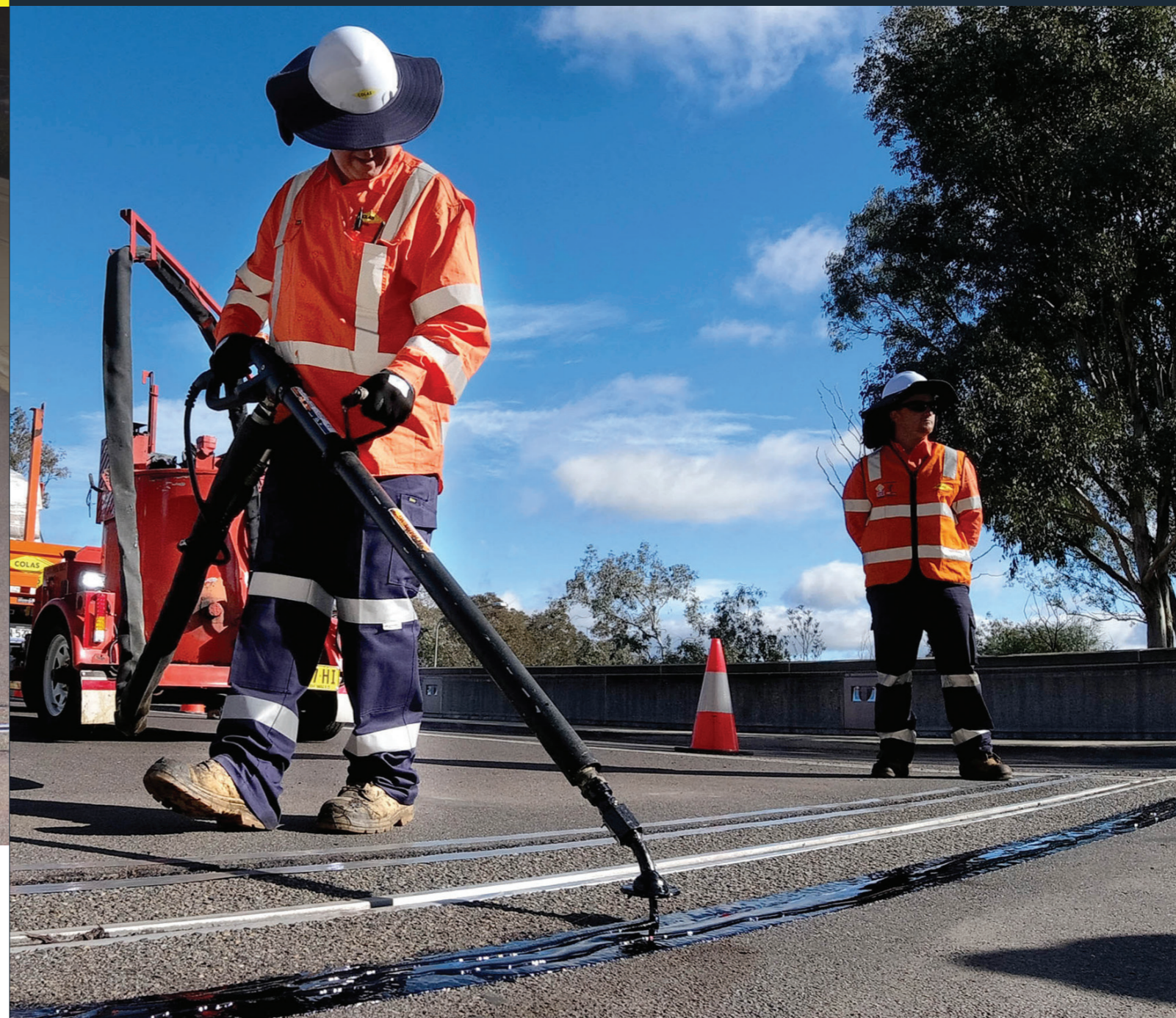
Crack sealing pavement maintenance at Parliament House
