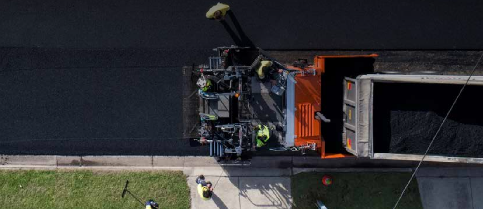
Paving low temperature Gap Graded Asphalt with crumb rubber
