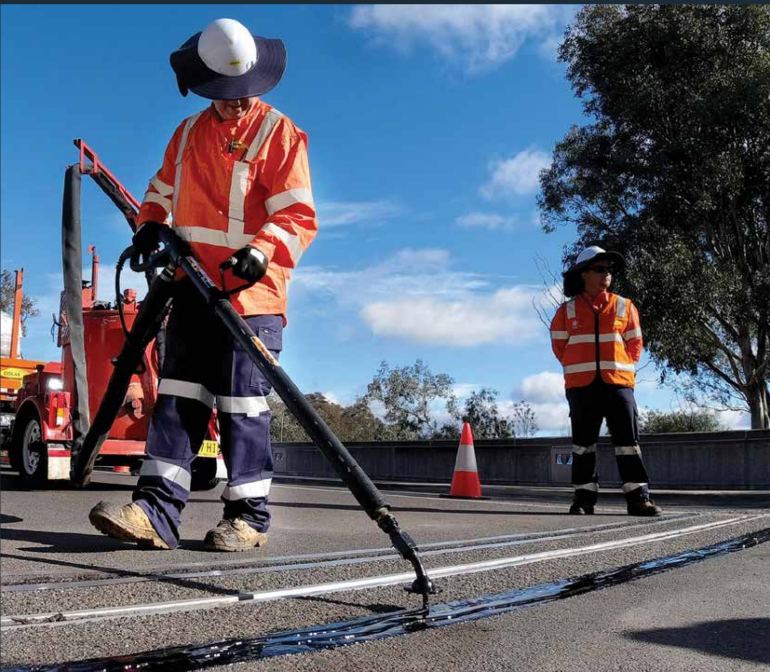
Crack sealing pavement maintenance at Parliament House
