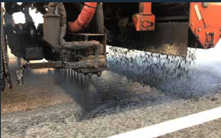
LV S15R being sprayed by the OB Vario synchronised sprayer and spreader
